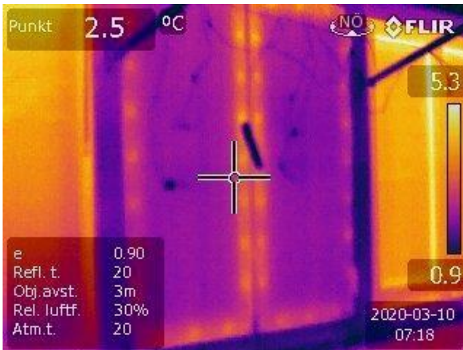
Exterior, the left side is painted with Thermoshield Extérieur and the right side is painted with Caparol Amphisilan. The position is southeast.
